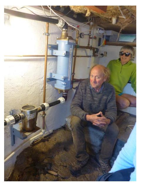
In this photo, Gus is showing Penny the sea-source loop, with the stainless steel filter and the heat exchanger (powder blue). The heat pump itself, in the cupboard behind Penny, looks pretty much like the back of a fridge!
